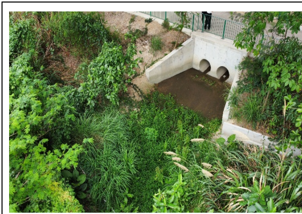
Photo No. 5 – Existing stormwater inlet under the elevated Heung Yuen Wai Highway from which the flow will pass through twin 900mm diameter drains and go to the west
